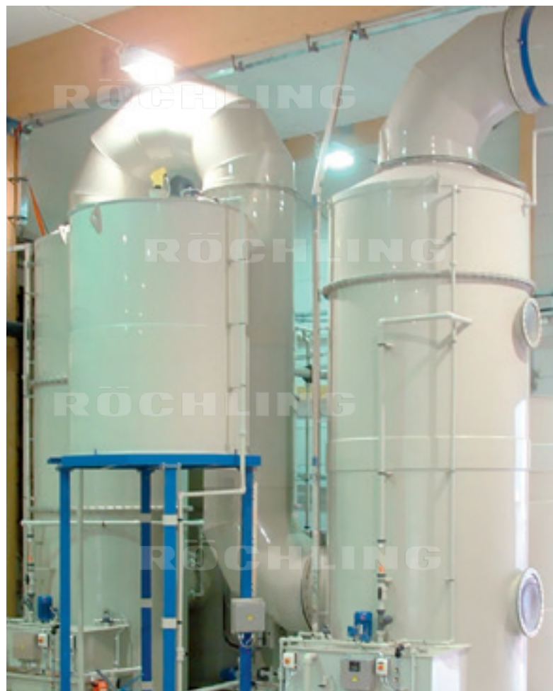
The liquids and gases used in exhaust-air cleaning plants are often severely corrosive. Thermoplastics are used here because of their special corrosion resistance.
