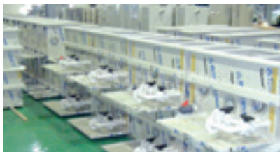
Polystone® P homopolymer grey Tank for a copper-coating plant
