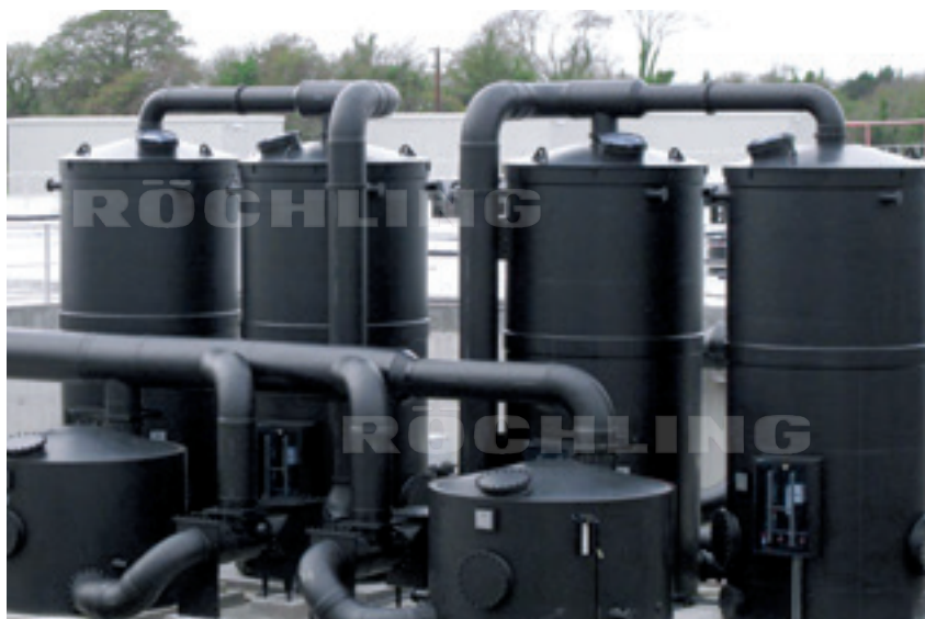
Polystone® G black B 100 Air purification system in a water treatment plant
